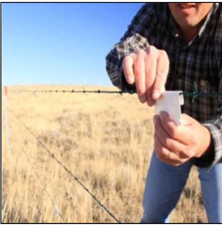
Figure 2. Installation of a fence marker.
